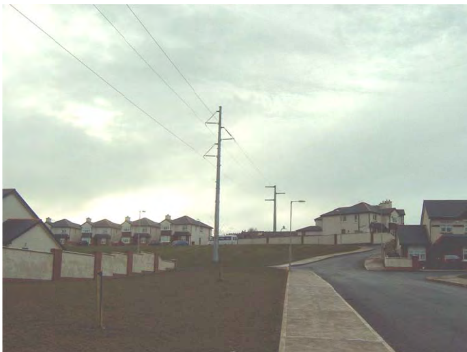
Photo 2: 110 kV Monopole Overhead Line in Cork
